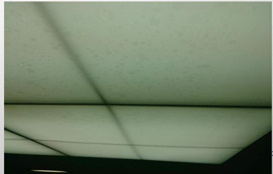
Microbial load in diffuser screens of a UDAF
